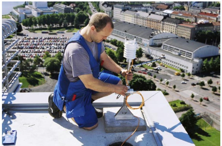
A WXT520 being installed at the top of the 72-meter tower at the Olympic Stadium in Helsinki, Finland.
